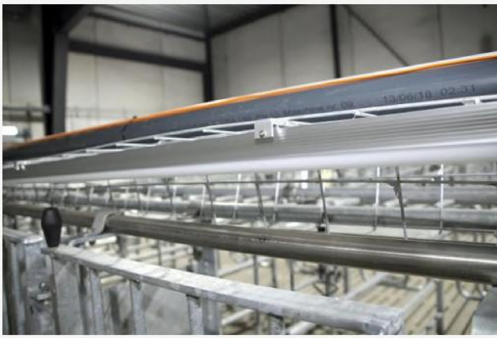
Investment has been made in LED lighting for the barn. Partly in the iolen, but lights have also been installed in front of everyone paddocks for better reproduction.
